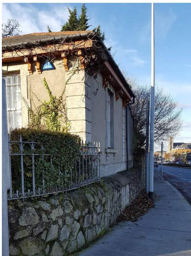
Figure 17.10 - New boundary wall
