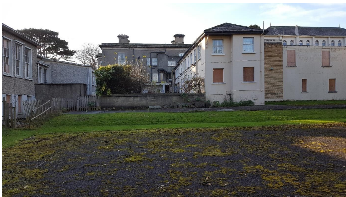
Figure 17.7 - View from North-east (pre-2021 demolitions)
