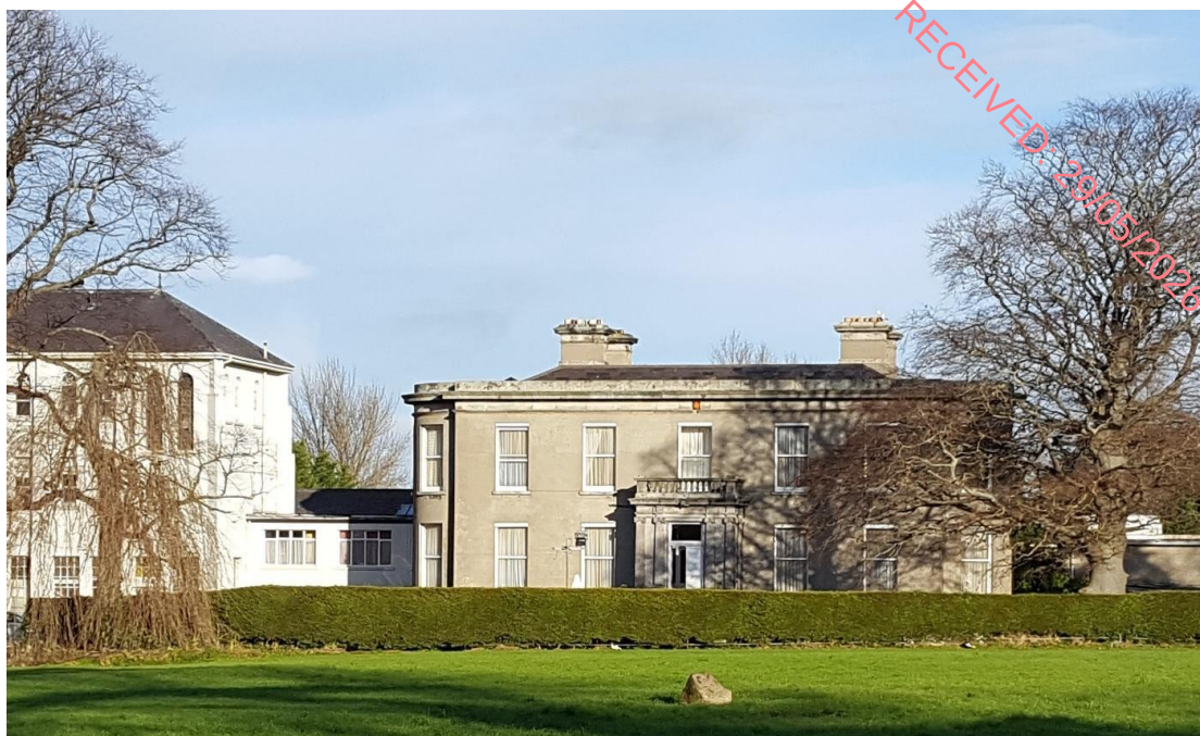
Figure 17.8 - View from South-west (pre-2021 demolitions)
