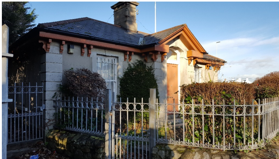
Lodge at St Teresa's House
