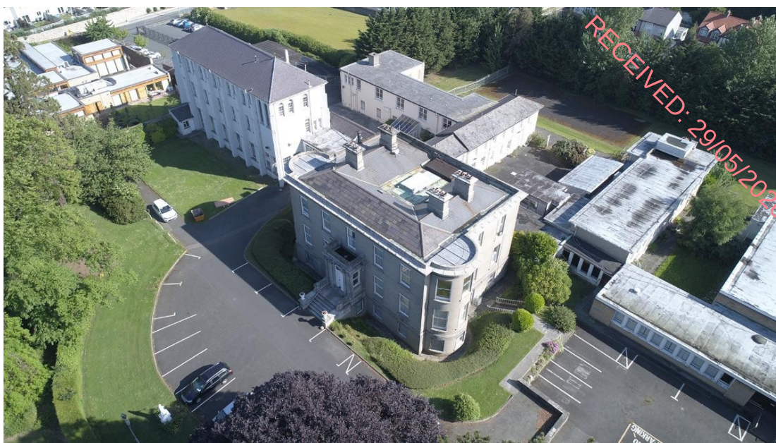
Figure 17.6 - Aerial view from South (pre-2021 demolitions)
